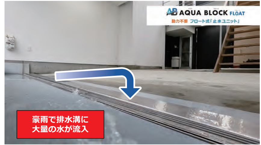
6 豪雨時、排水溝へ大量に雨水が流入 During heavy rains, a large amount of rainwater flows into the drains. 排水管がオーバーフローを起こし、排水溝に雨水が溜りだす Drainage pipes overflowed and rainwater collects in the drains.
